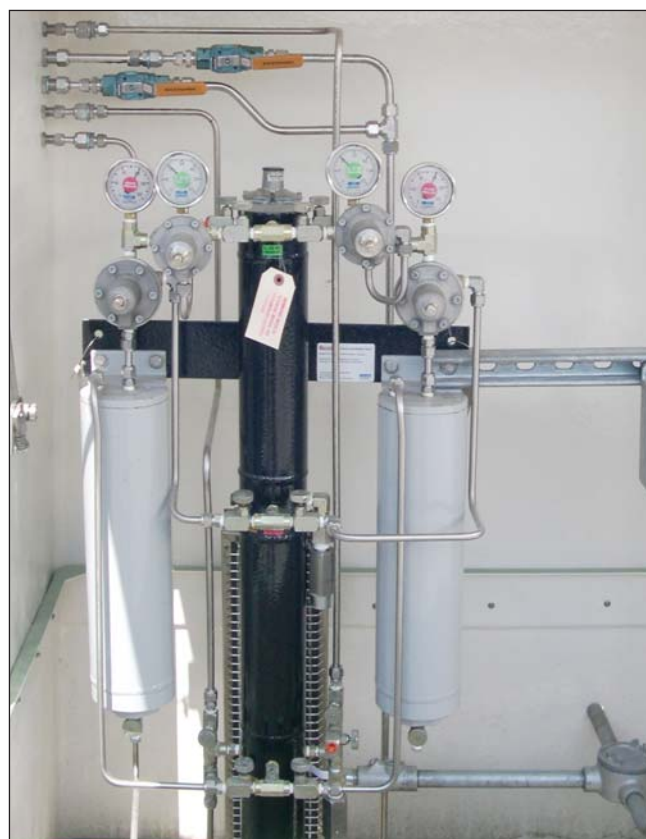
Figure 8 - Single PIC Installed in Becker CAB Series Fiberglass Enclosure
