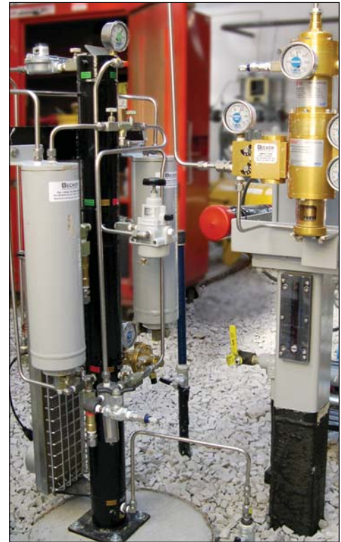
Figure 9 - PIC Installed Inside Pressure Limiting Station Building
