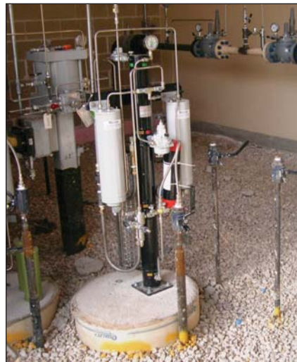
Figure 2 - PIC Installed Inside a Natural Gas Regulation Facility
