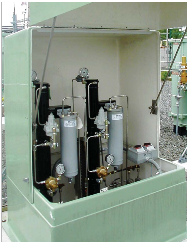
Figure 7 - Dual PICs Installed in Becker CAB Series Fiberglass Enclosure
